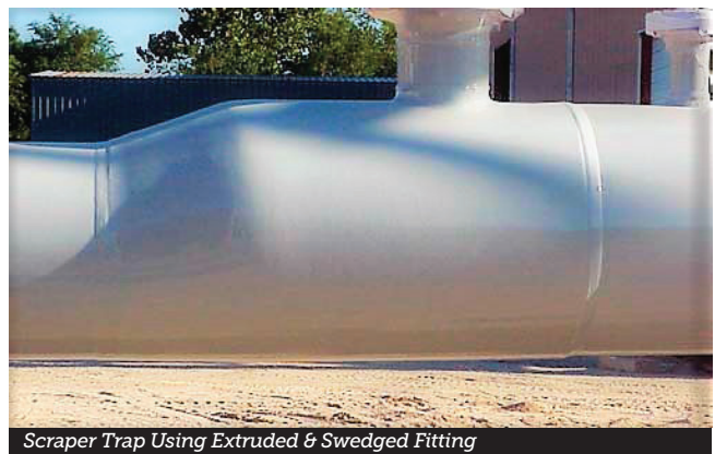
Scraper Trap Using Extruded & Swedged Fitting
